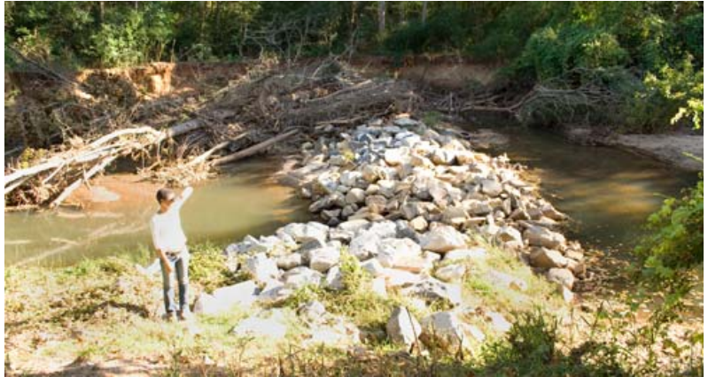
Rock Dam on South River
